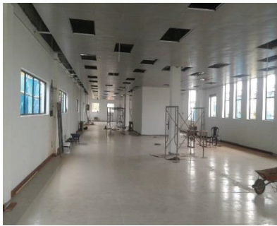
Construction of four storied stores complex
